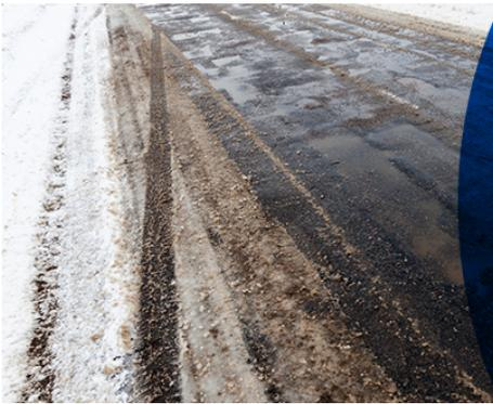
The best way to spread salt as a de-icer is to **remove as much snow as possible** before application.
